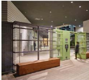
FENCE WITH LOW IRON GLASS INFILL PANELS
