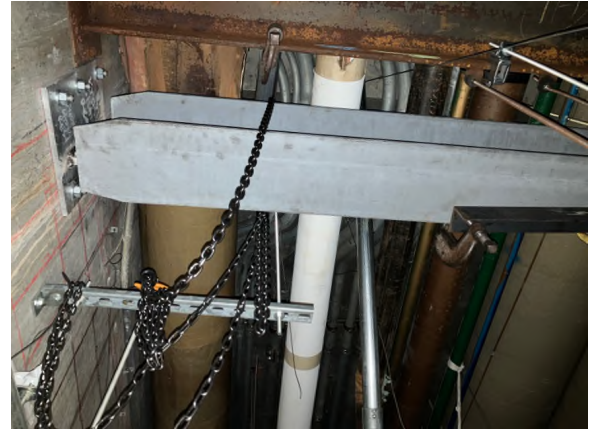
New MEP Utility Support Beam and Seismic Supports
