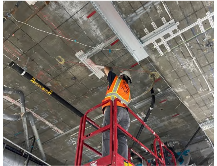
Top Track Installation
