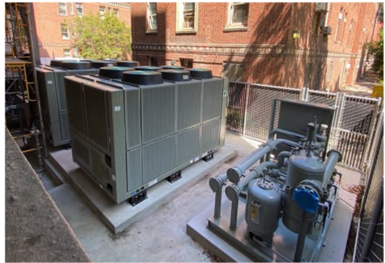
New Mechanical Chillers Installed
