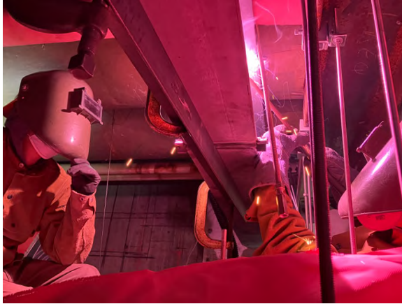
New MEP Utility Support Beam and Seismic Supports
