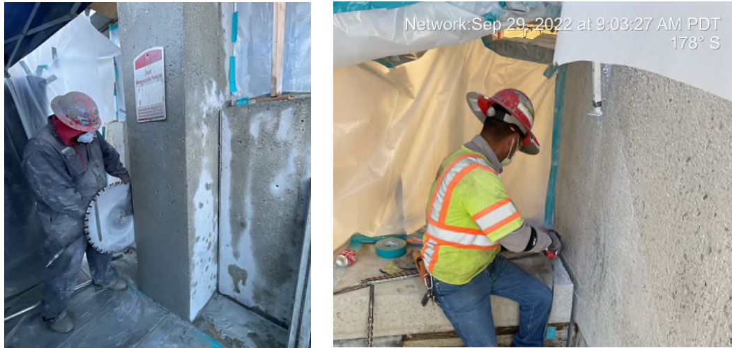
Exterior sawcutting at spandrel locations
