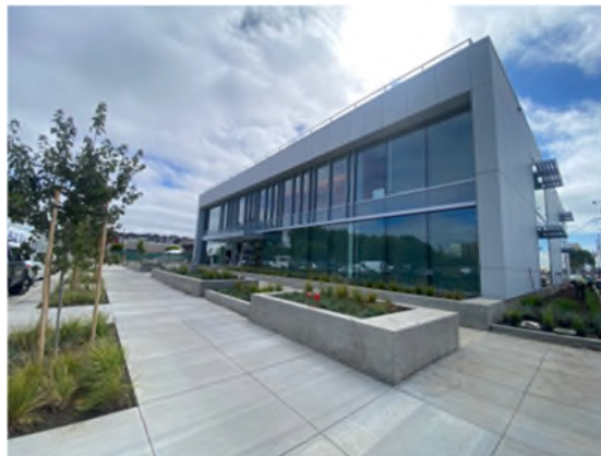
S/W View of Building
