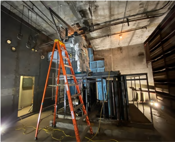
Existing AHU Removal
