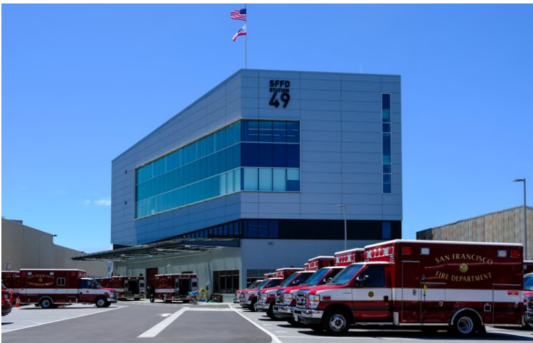
Front of New SFFD Station 49
