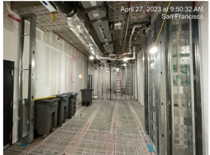
3 rd Flr - Framing at the Repair Room
