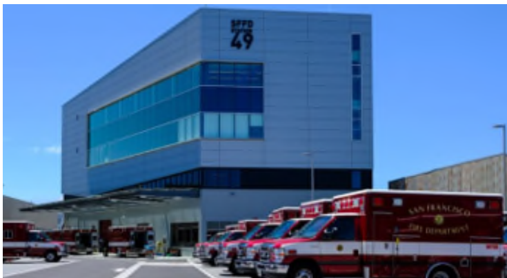
Ambulance Deployment Facility
