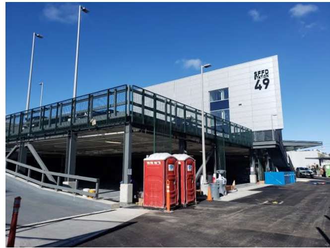
View of backside of the new SFFD Station 49 and upper garage deck.
