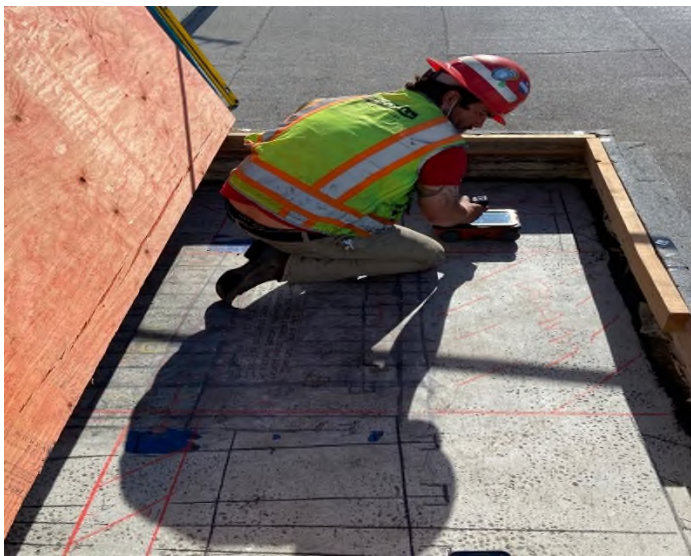
Roof Scanning for new Mechanical Equipment Platform
