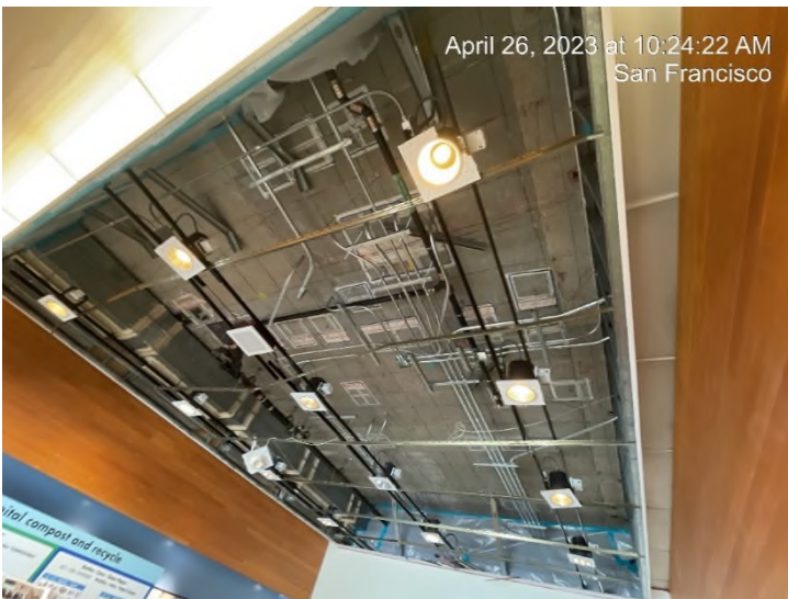
2 nd Flr - Plumbing and Electrical Conduits Below Nurse Station
