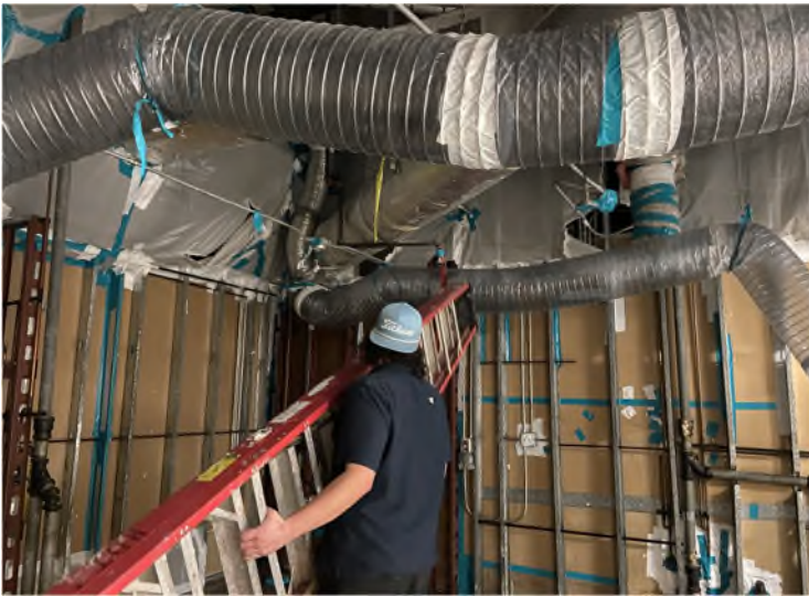
Tracing Conduit in the Shower Room
