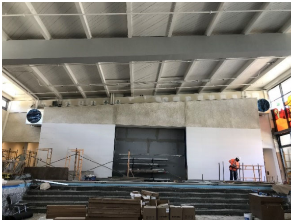
Construction Photo, October 2019
