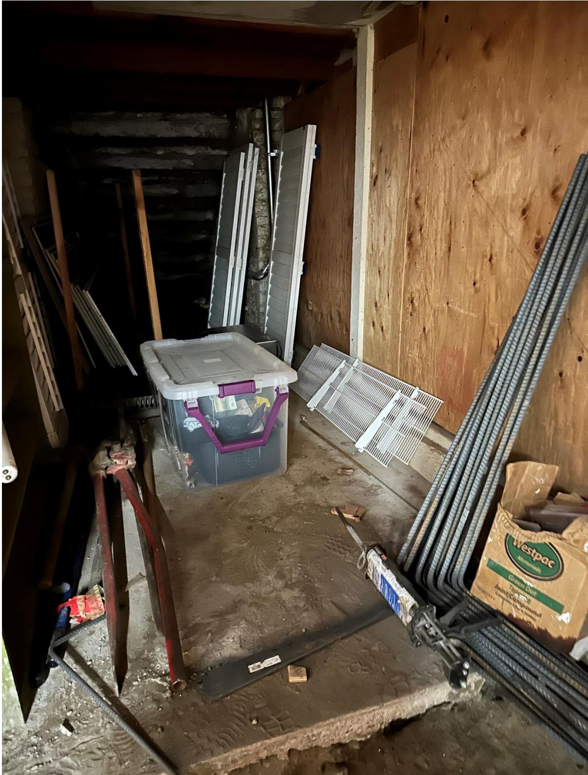
Photo 1: North side looking into crawl space underneath entry stairs
