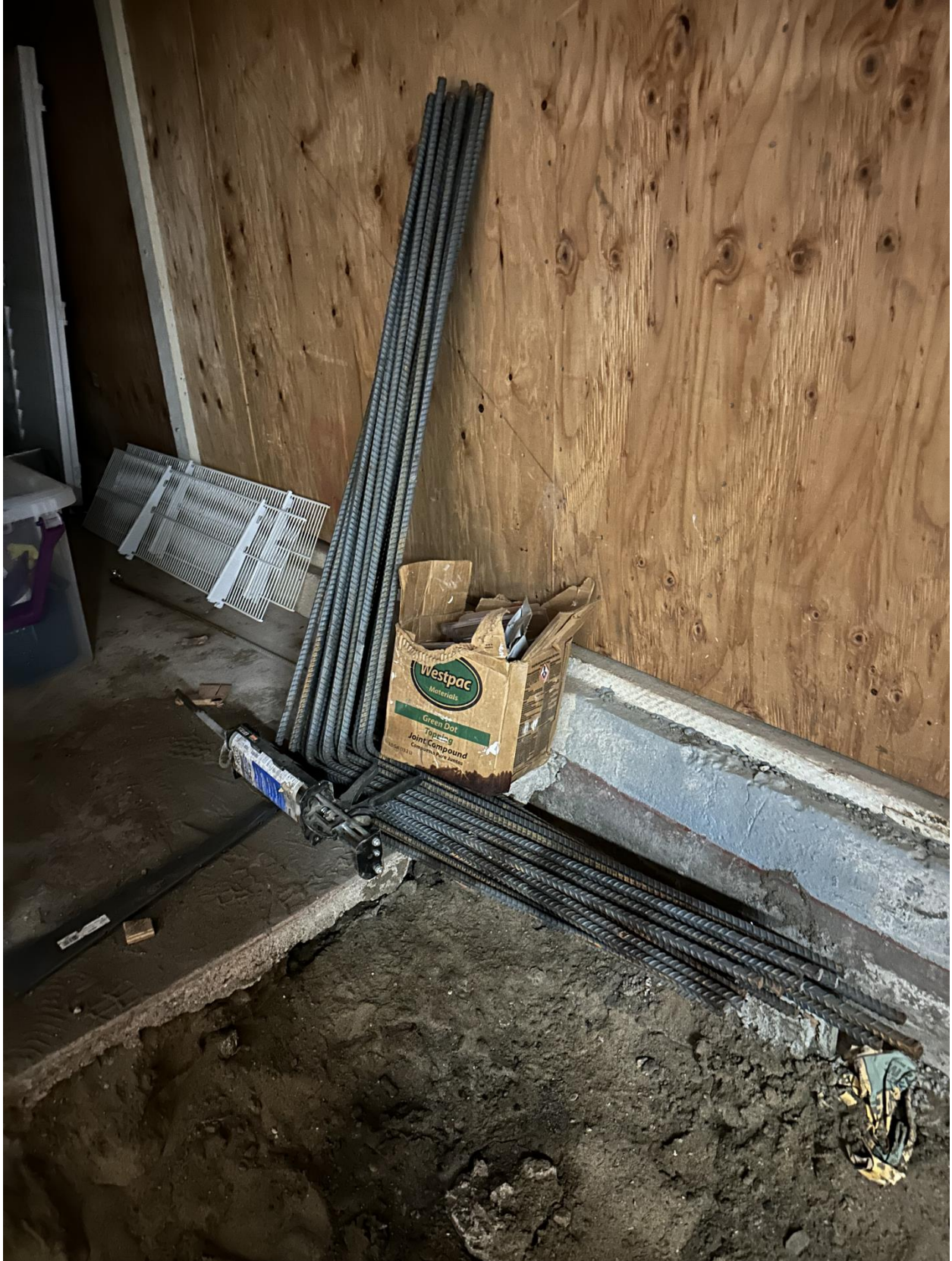
Photo 2: North Side Interface at (E) Garage Slab and Excavation
