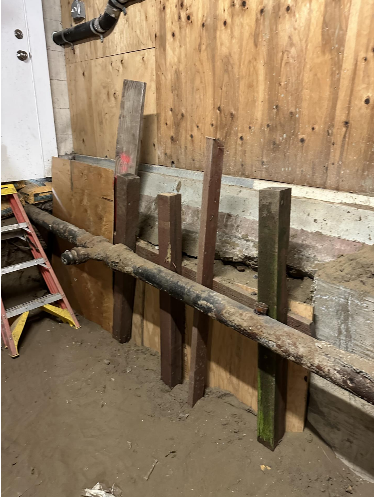
Photo 13: South East Corner
