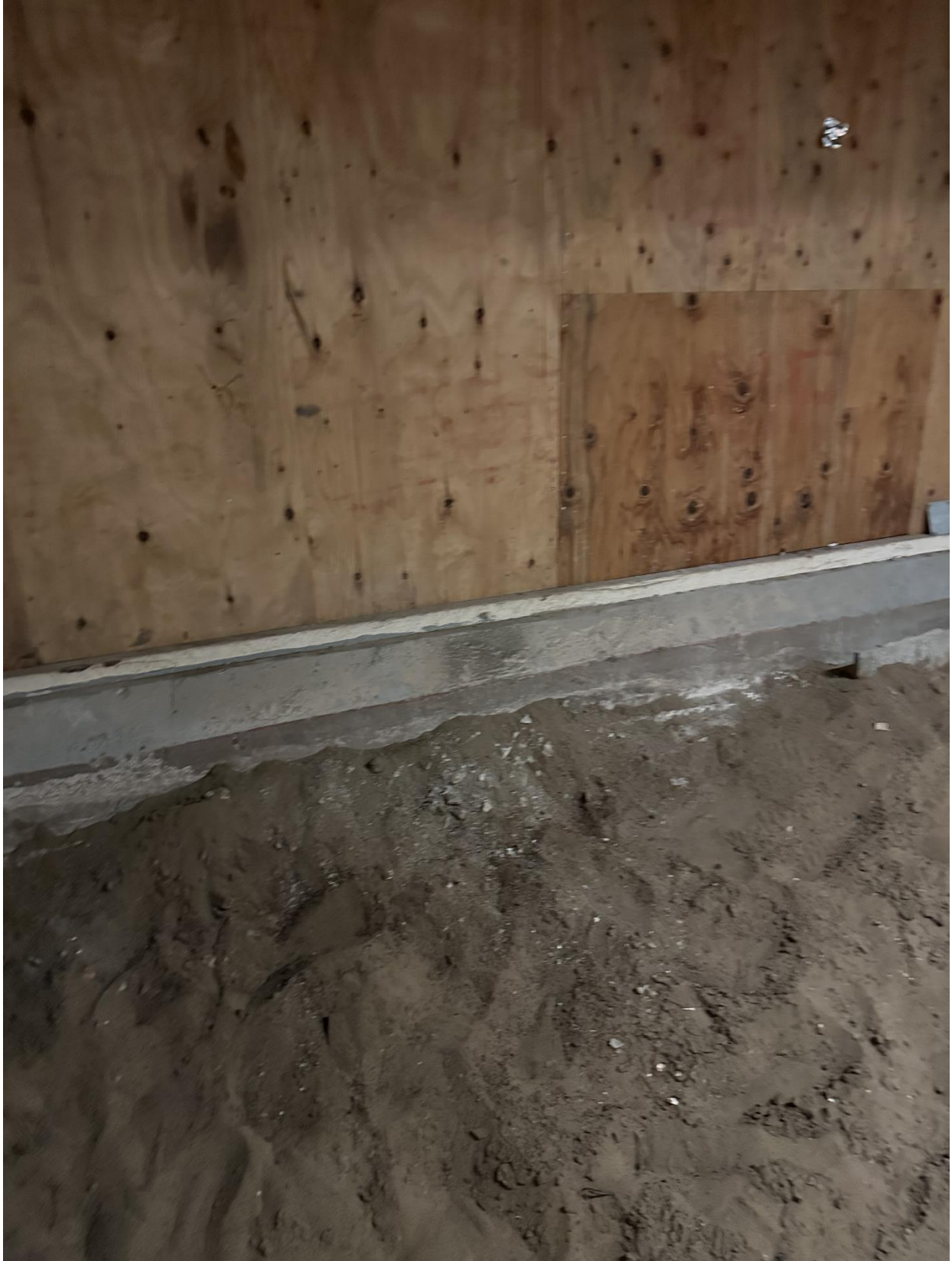
Photo 5: North Side: Backfilled Excavation at Northern Property Line
