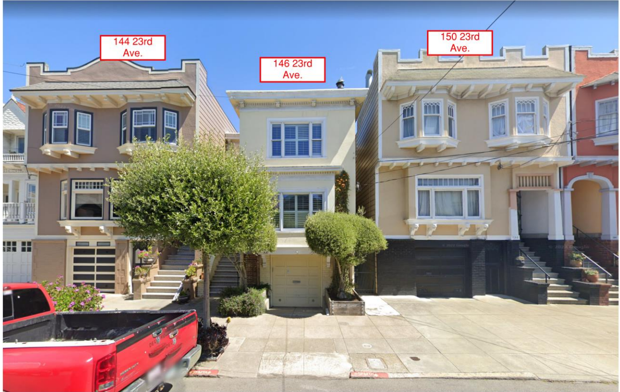
Figure 1: Street View of Subject Property and Neighboring Buildings
