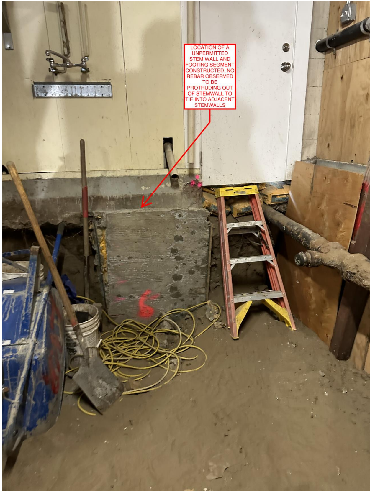
Photo 11: South East Corner
