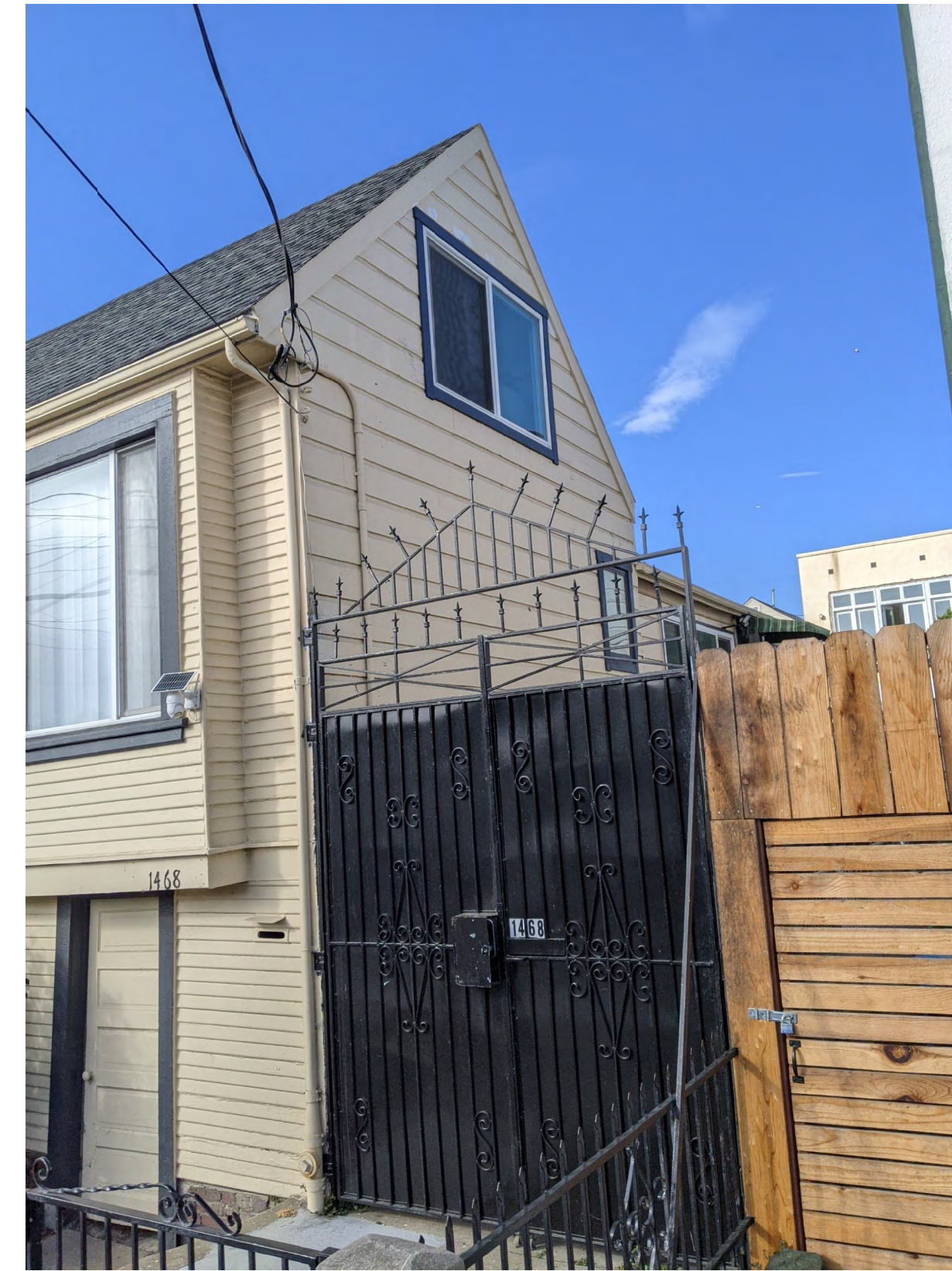
2-NEW FRONT SECURITY METAL GATE
