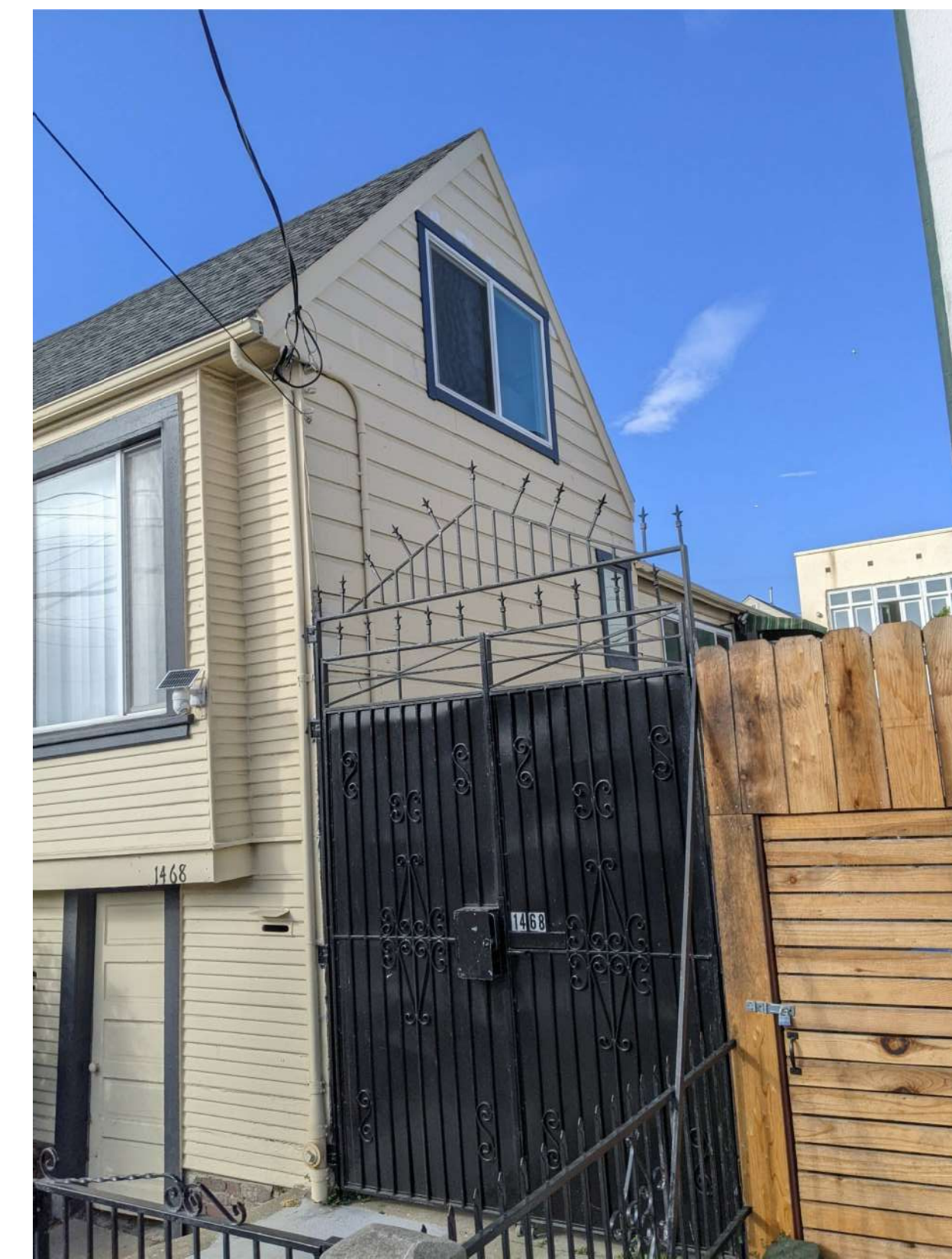
2-NEW FRONT SECURITY METAL GATE
