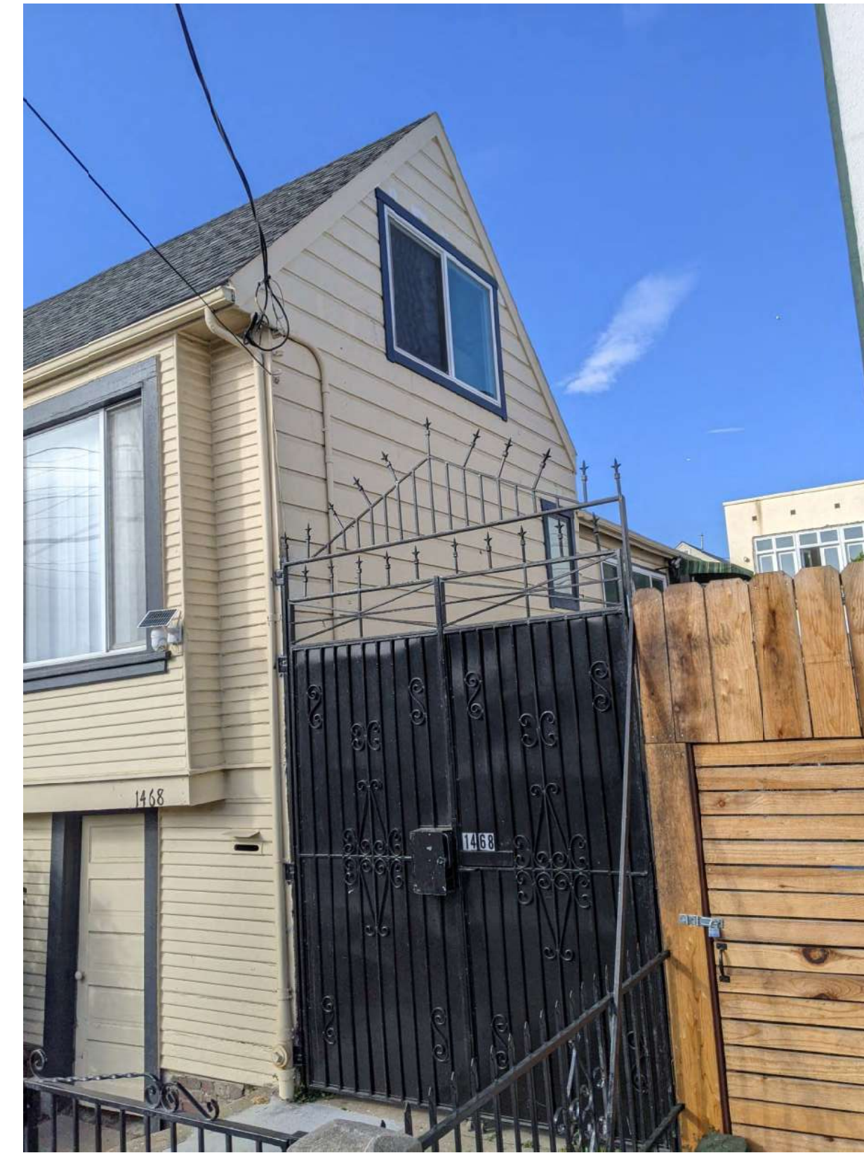
2-NEW FRONT SECURITY METAL GATE
