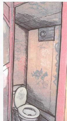
Bathroom is too small for a wheelchair to turn around, and is missing fixtures and grab bars
