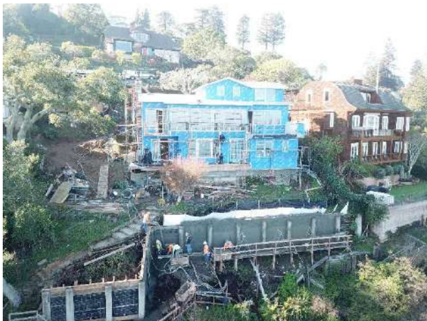
312 Beach Road, Belvedere, CA Project Type: Residential Construction Design of retaining walls, landscape features, and ADU on a steep site in Belvedere.
