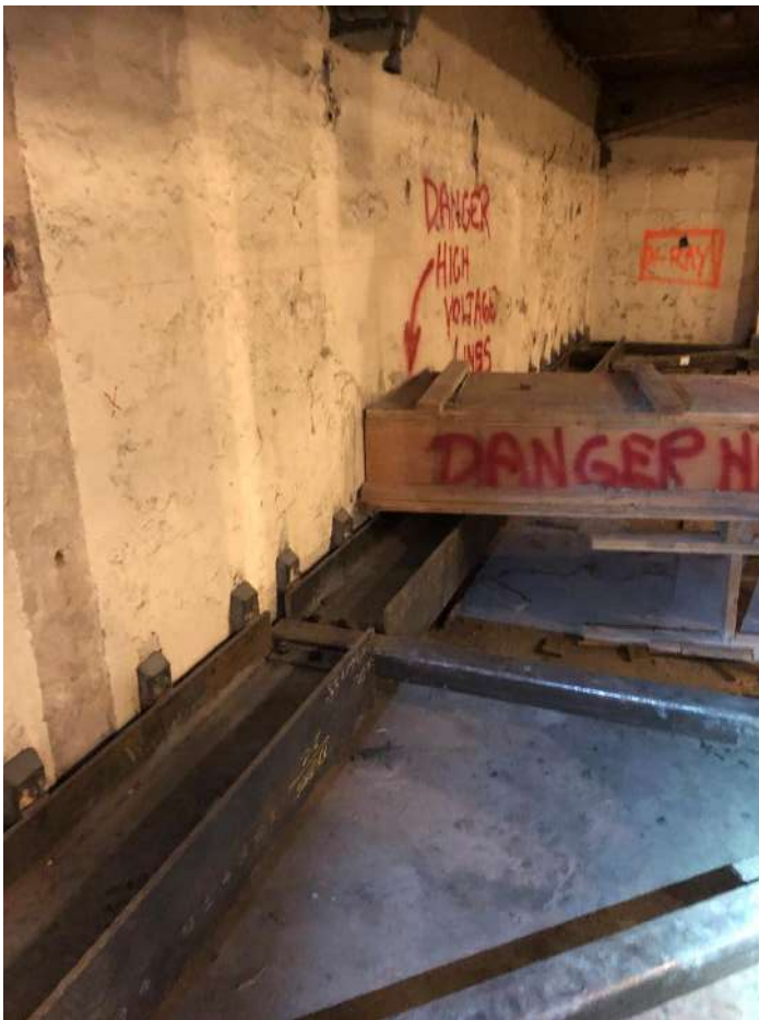
419 South Spring Street, Los Angeles, CA Project Type: Commercial Earth Shoring Basement excavation shoring for seismic retrofit of existing building in Los Angeles. Scope included design of earth shoring, coordination with contractor and various sub-contractors, LADBS and BOE responses.
