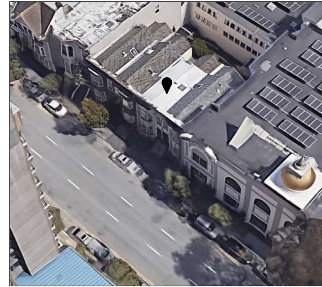
1. AERIAL PHOTO FRONT OF PROPERTY LOOKING SOUTH-EAST
