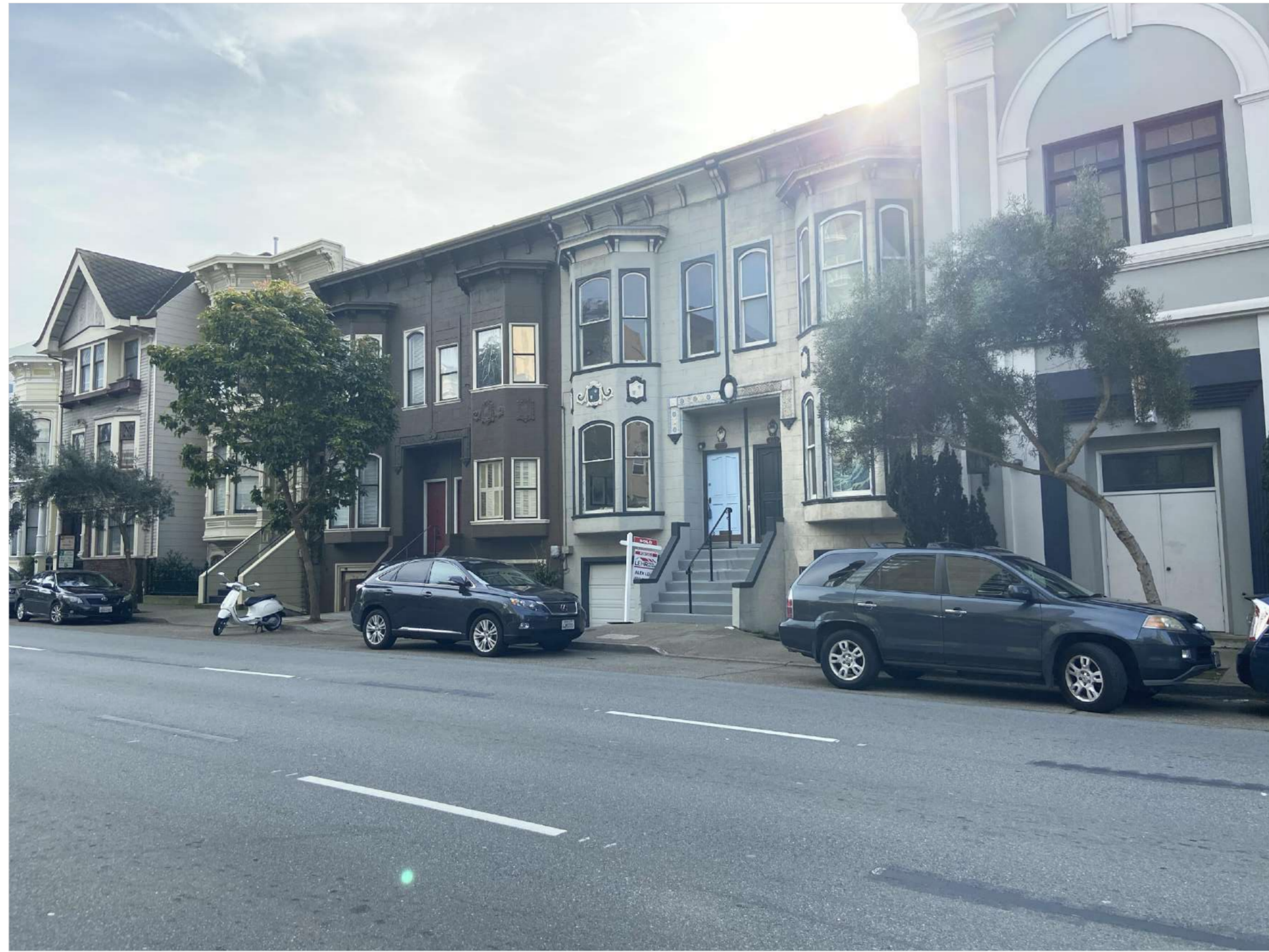
1 FRONT LOOKING SOUTH EAST
