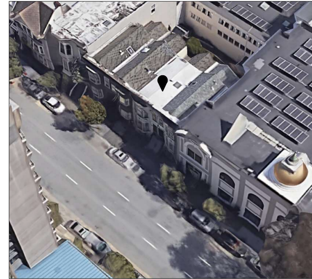
1. AERIAL PHOTO FRONT OF PROPERTY LOOKING SOUTH-EAST
