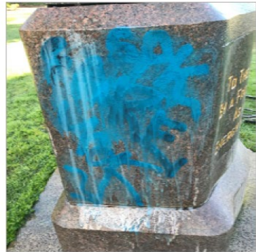
Figure 42: Detail during the application of paint removal products.
