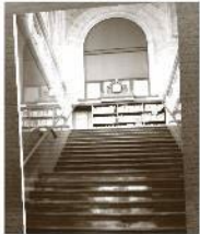
Original stairs and window
