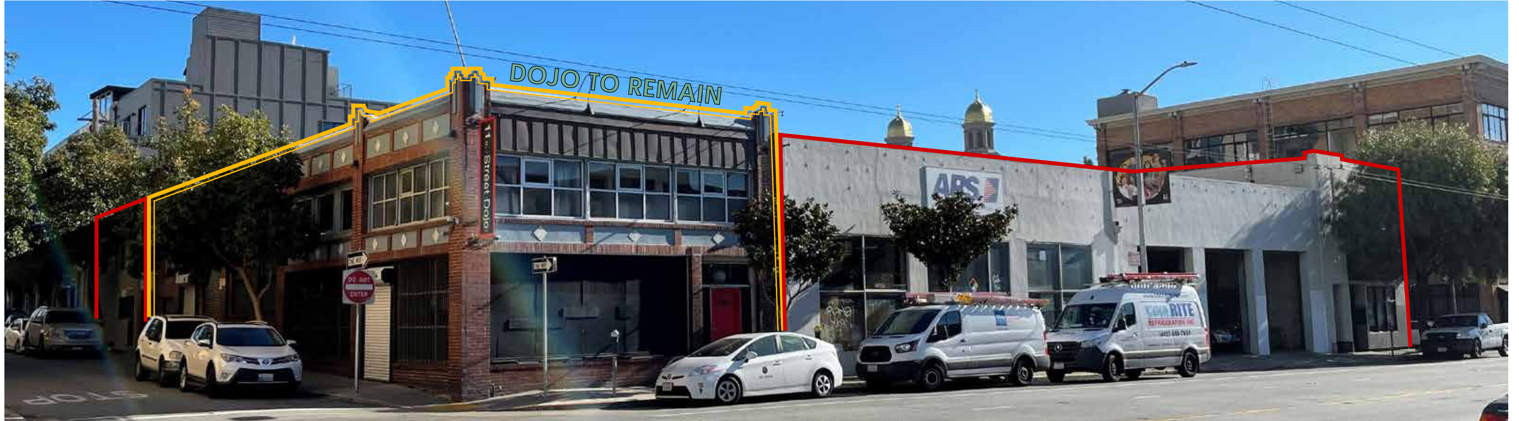
11 th ST LOOKING NORTHEAST
