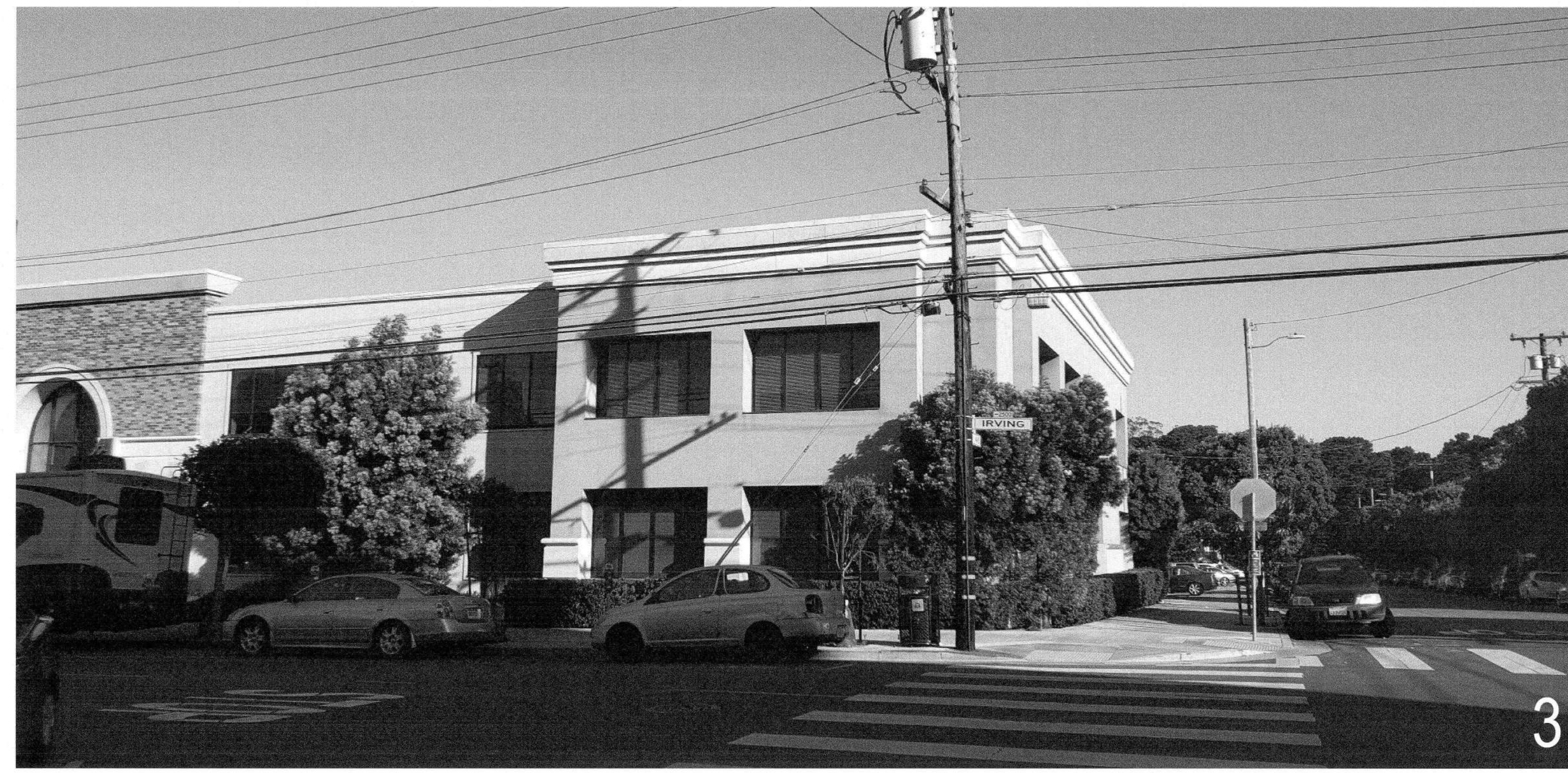
26TH AND IRVING LOOKING NORTH
