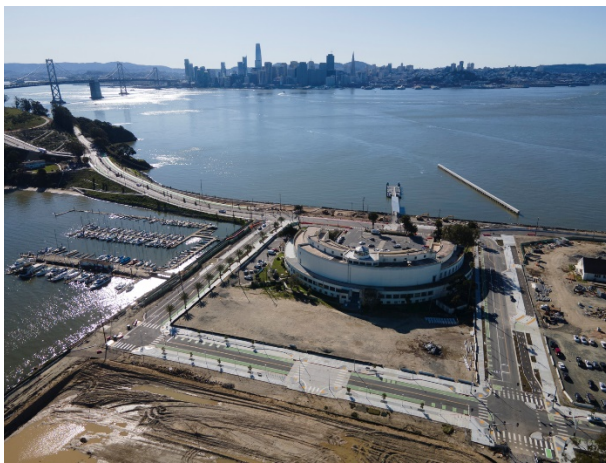
View of the Treasure Island Administration Building and leveled Parcel B, image by Andrew Campbell Nelson
