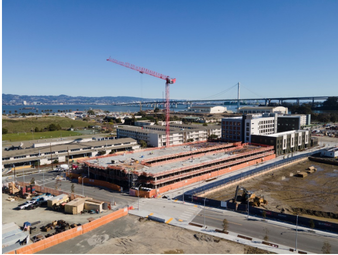
Star View Court construction progress, image by Andrew Campbell Nelson
