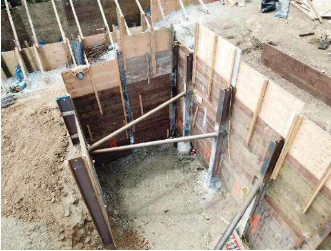
323 Cumberland Street, San Francisco, CA Project Type: New Residential Construction Design of temporary earth shoring for building excavation and complete foundation installation.
