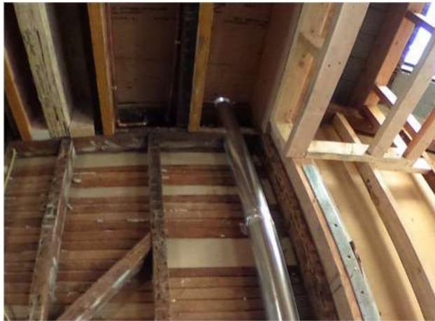
Photo 2: A New Vent Line installed at the Shared Property Line Bearing Wall
