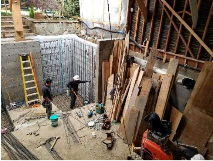
2625 Scott Street, San Francisco, CA Project Type: Residential Construction Design of temporary earth shoring for building excavation, complete foundation installation, and full building renovation. Project shoring consisted of sectional pit construction with concurrent house shoring.
