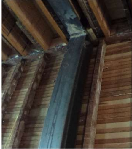
Photo 3: A new Steel Moment Frame Column installed in the plane of the Shared Property Line Bearing Wall
