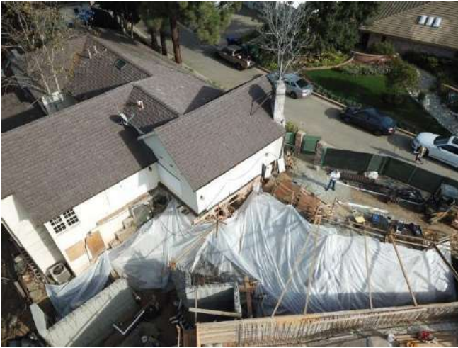
357 Crown Drive, Los Angeles, CA Project Type: Residential Addition Design of temporary house shoring for adjacent building excavation.
