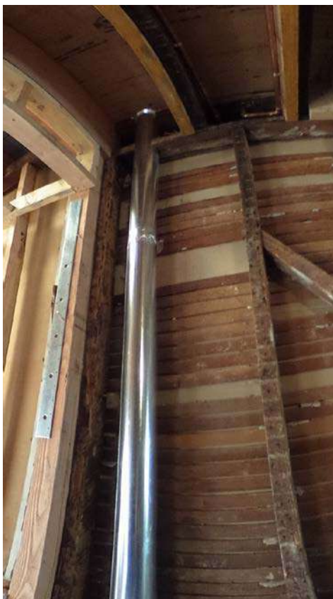
25 2: New flue installed in party wall 26 without permits 27
