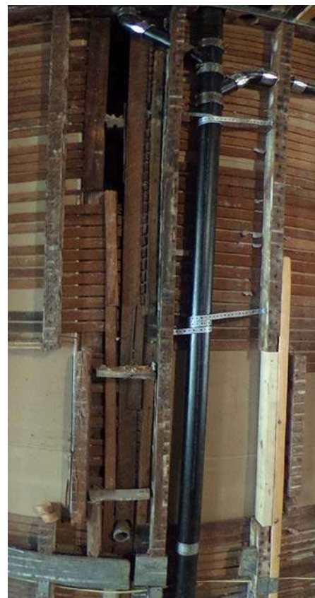
28 1: New plumbing pipes and electrical installed in party wall without permits
