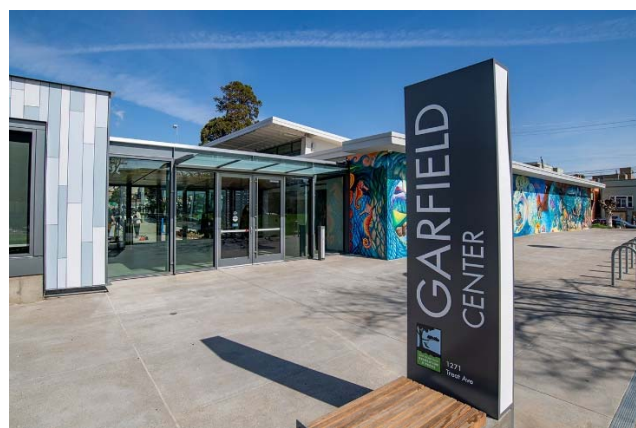
Project Complete, April 2021
